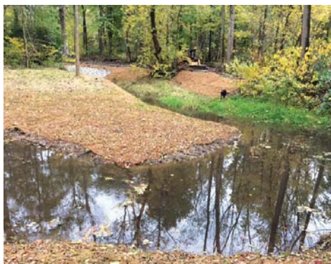
Dillon Creek embankment enhancement for sediment control
