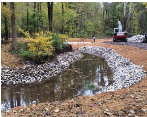
Dillon Creek sediment and erosion control work upstream
