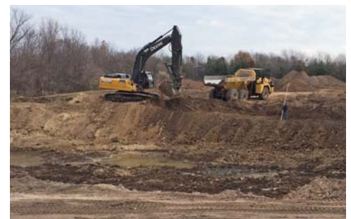
Thorpe Basin Construction
