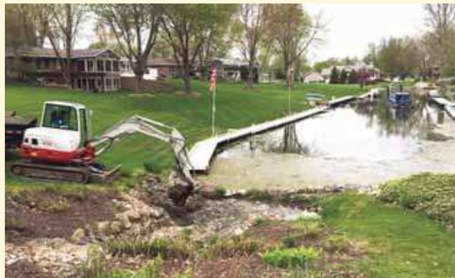
Sediment Basin clean out is Martin Creek into Leeland Addition
