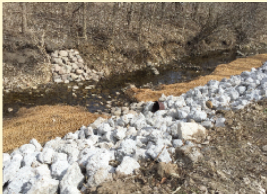
Turkey Creek Tributary stream stabilization
