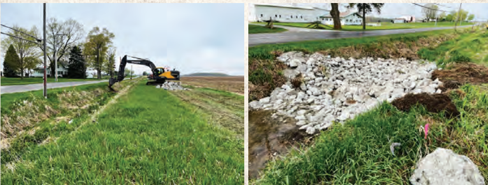
Dillon Creek Branch Work – creating riffles in the Branch
